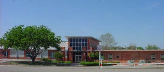
The front of Comal Elementary building, as seen from FM 482.
